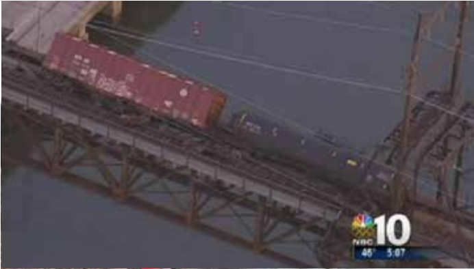
A catastrophe was narrowly avoided in Philadelphia when six tank cars derailed on a rail bridge in January 2014
